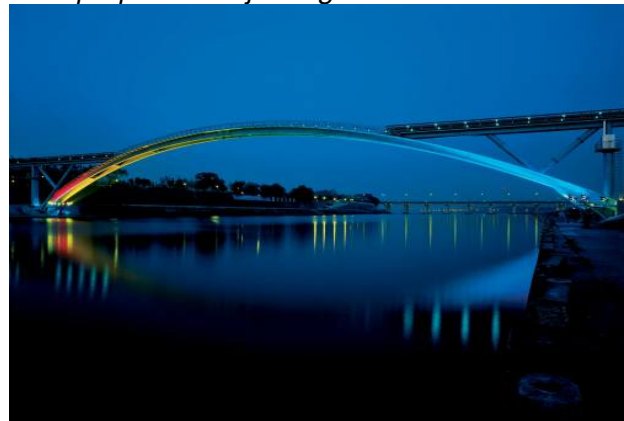
Footbridge of Peace in Seoul built using Ductal® RudyRicciotti Photo: Philippe Ruault
